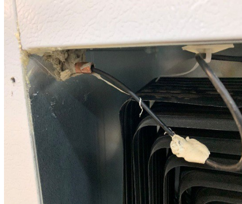
Sensor probe with bulbwell foamed
