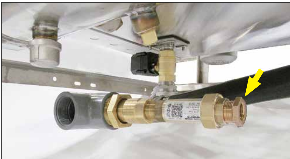
Fig. 7 - Mechanical DWT Valve
