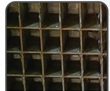
Grid is difficult to clean. A dirty evaporator can cause diminished production, increased service cost and premature equipment failure.
