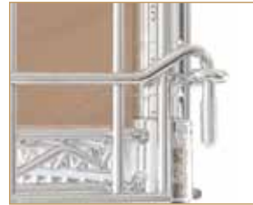
Protective cover on exposed wire ends.
